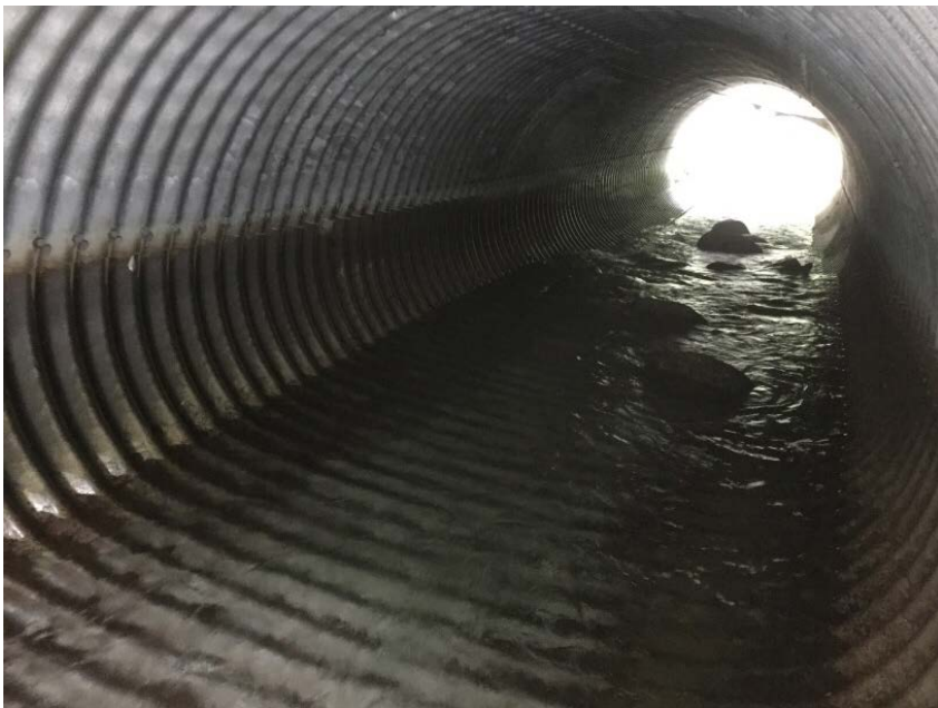
Looking through culvert from inlet
